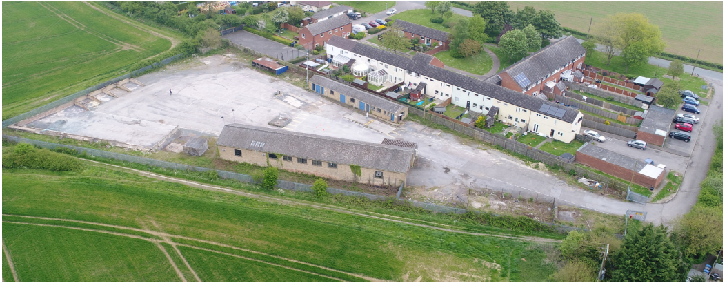
The site just before demolition
